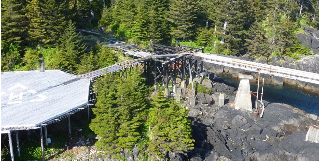
Figure 1. Helipad, tramway, boathouse foundation and pier (left to right).
